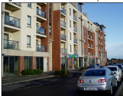
Figure 3.10: Main St units off Belmayne Ave
